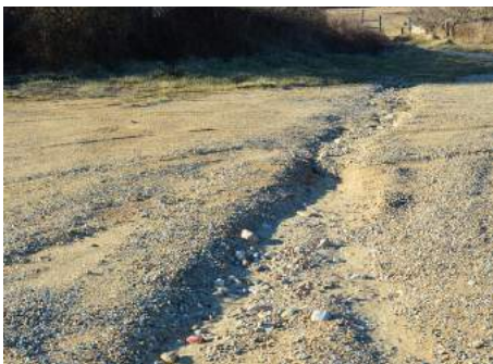
Concentrated stormwater leads to heavy erosion along paths(left) and in the beach parking lot (right). The erosion makes walking hazardous and drives up maintenance costs.
