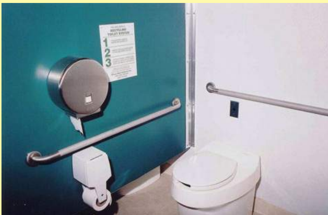
Composting toilets look similar to conventional toilets, but care should be taken to educate visitors on what can and cannot go into the toilets. (Credit: Clivus New England Inc.)
