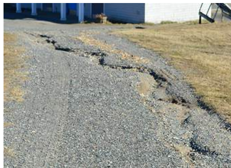
Concentrated stormwater leads to heavy erosion along paths(left) and in the beach parking lot (right). The erosion makes walking hazardous and drives up maintenance costs.
